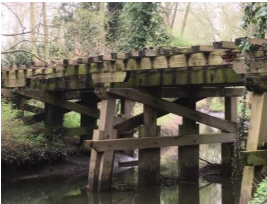
Photo 15: Historic Trestle Bridge
