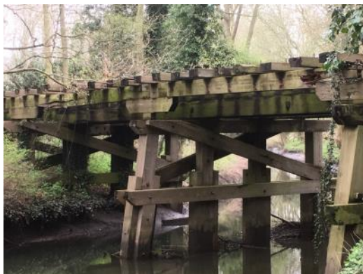
Photo 1: The Trestle Bridge
