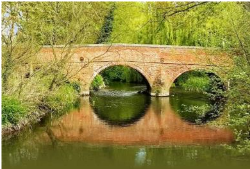
Photo 9: Blue Mills Bridge over the River Blackwater
